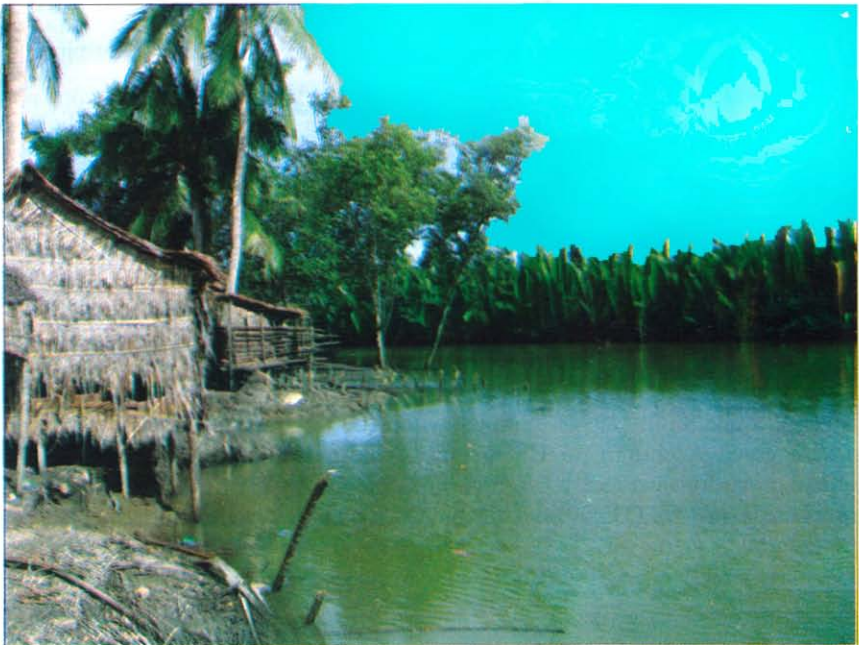
Photo 2 Protection of embankment erosion by mangrove trees in Tebinseik Village (Although residential areas were eroded by the tidal wave in the left-front, the area located in the back central part of photo was protected by presence of Thame trees)
